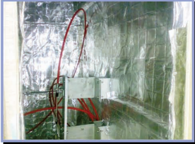
A60 plastic penetrations on bulkhead by UNICOLLAR®
