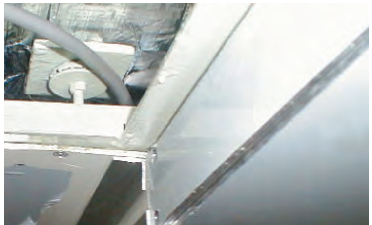
Installation of detail above using QuietClad with available polar white acrylic finish aboard a 45M power yacht. Sheets are supplied with a removable protective film (shown peeled away at edges) to prevent marring of finish surface.
