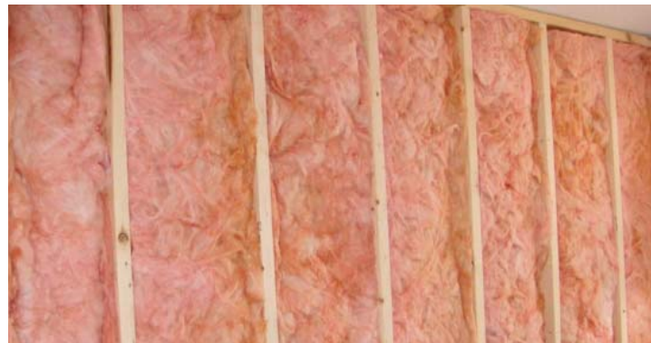
Acoustic Fill in between studs of privacy wall
